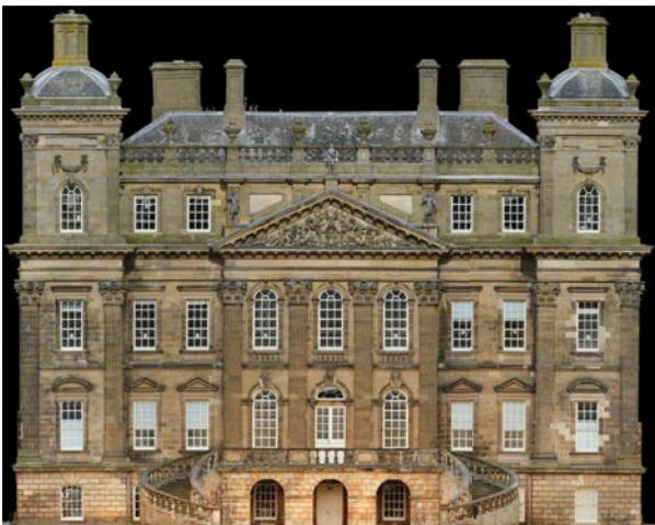
Figure 1. Orthophoto for the entire front elevation of Duff House.
